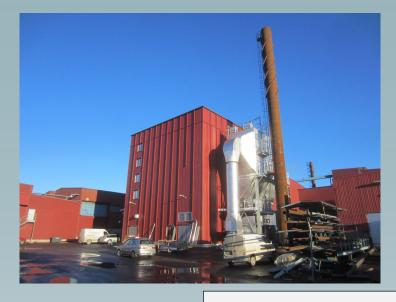
Saxwerk have delivered a 16MW boiler plant to Martinsons Trä AB for their kilns at the saw mill.
